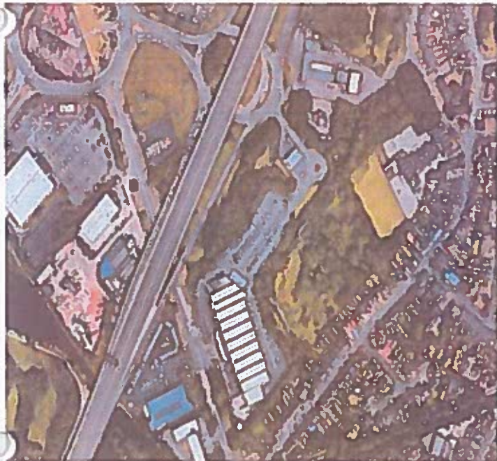
An aerial view showing the woodland where the development is proposed. Photo: Google Maps
